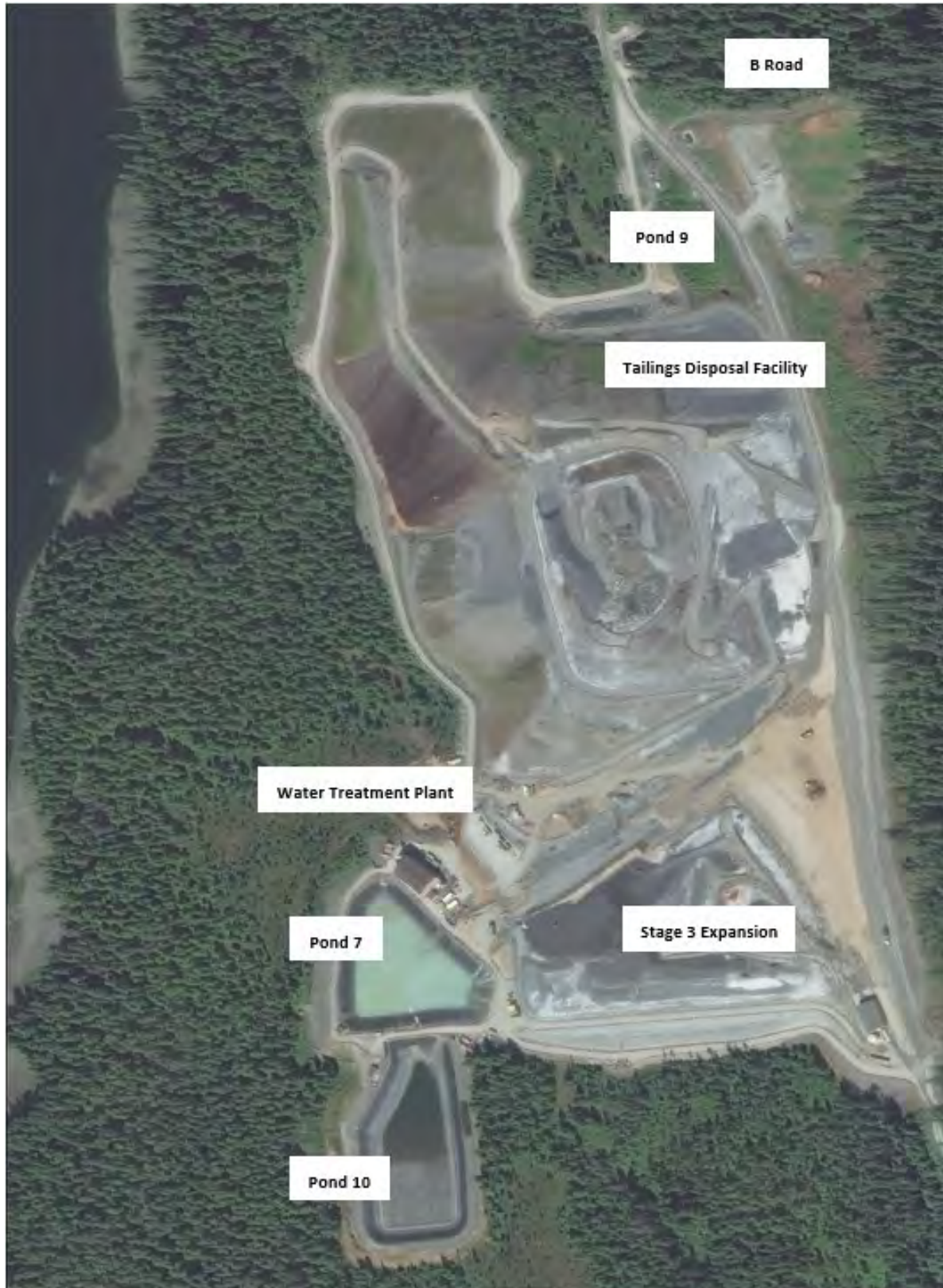
Figure 15-6: Hawk Inlet Dry Stack Tailings Disposal Facility
