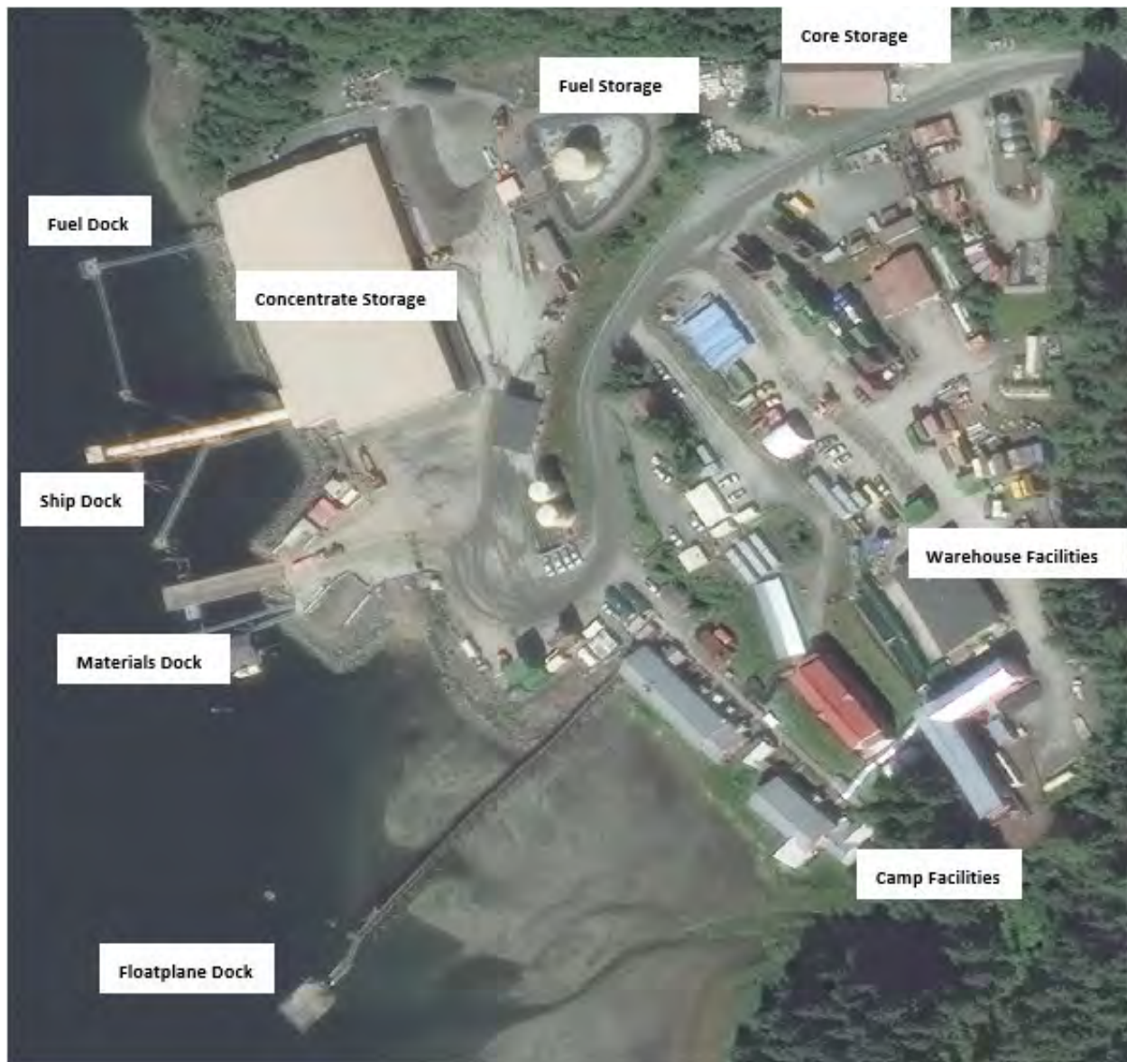
Figure 15-2: Hawk Inlet Infrastructure
